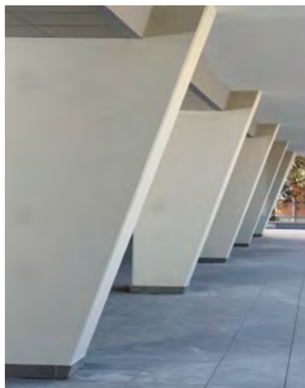
POSA SOPRAELEVATA / ELEVATED FLOOR INSTALLATION
