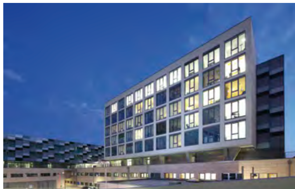
POSA SOPRAELEVATA / ELEVATED FLOOR INSTALLATION
